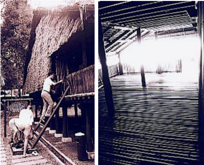
Figure 19: Traditional house from Sarawak, Malaysia. The house is placed on stilts and is made from bamboo allowing high rate of natural ventilation.
