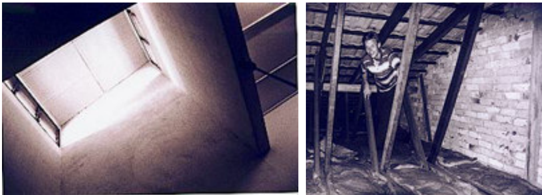
Figure 12: 1) Air-shaft in terrace house. The louvers are open at the top of the shaft for removal of hot air by natural ventilation. 2) No insulation or radiant barrier (aluminium foil) is usually found on the attic; this house is an exception (Serdang, Malaysia).
